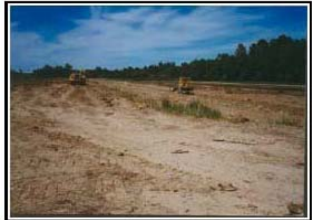
Figure 7-2: Wetland During Construction
