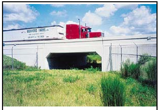
Figure 7-4: Example of Wildlife Crossing Under Highway
