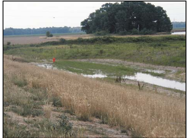
Figure 5.12-1: Sedimentation Basin BMP on Roadway Construction Project
