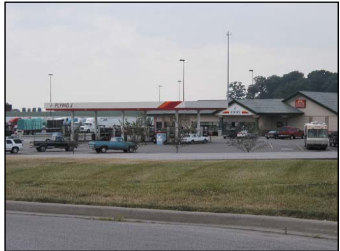
Figure 5.16-2: Typical UST facility
